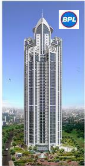
Premium Luxury Apartments Mantri Pinnacle (Installation Job).
