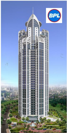
Premium Luxury Apartments Mantri Pinnacle (Installation Job).
